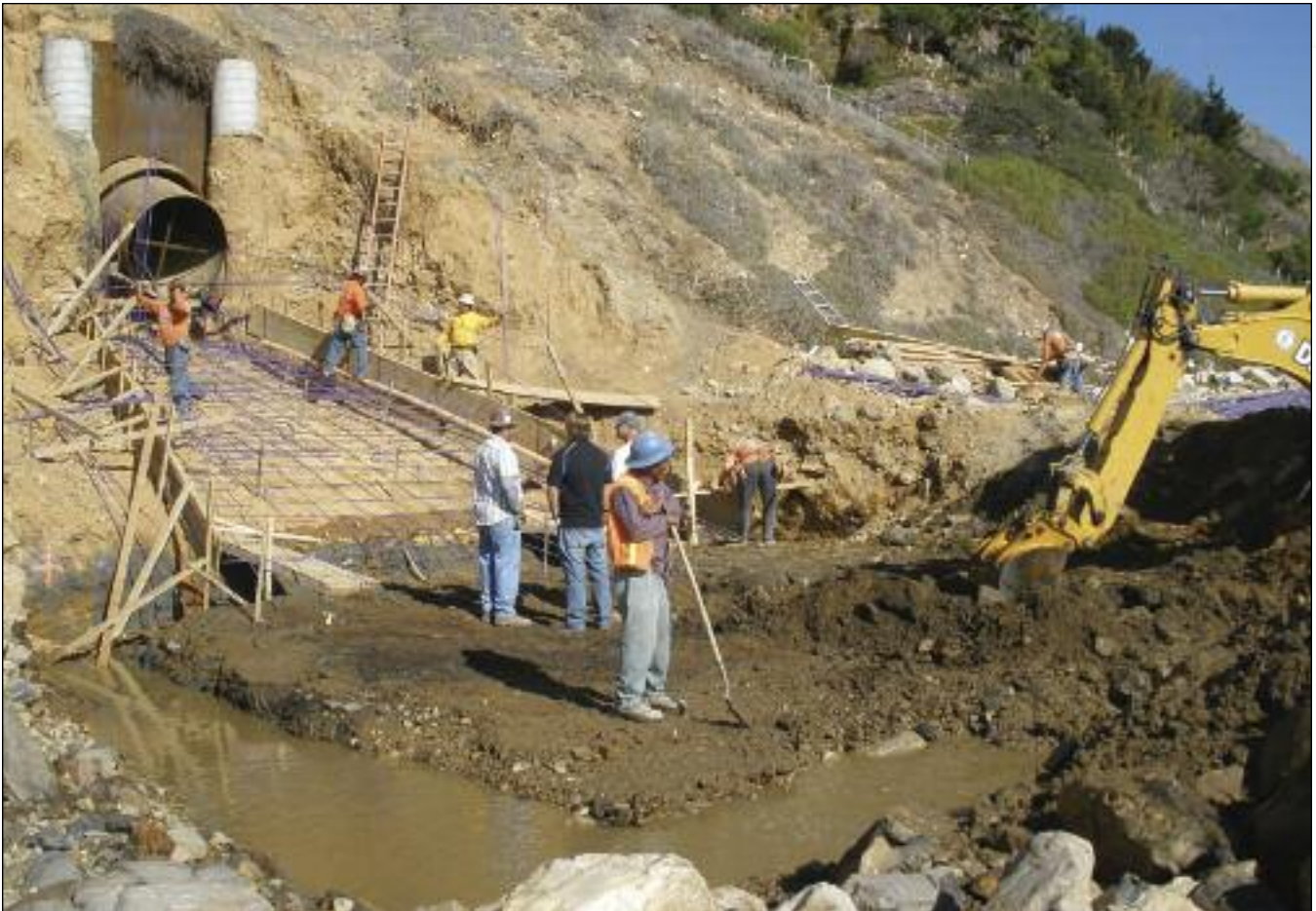
Outlet structure under construction with 24-inch-diameter soldier piles visible
