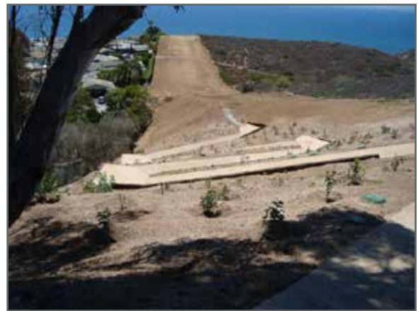
Figure 19. Completed maintenance access to the beach below 25th Street/PVDS.
