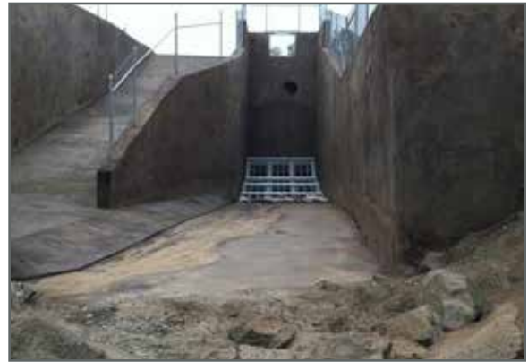
Figure 6. Completed upstream inlet structure.
