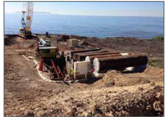
Figure 9. Lower tunnel launch pit 150-feet above the Pacific Ocean (with Catalina Island beyond).
