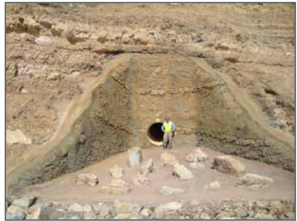
Figure 18. Outlet structure completed.
