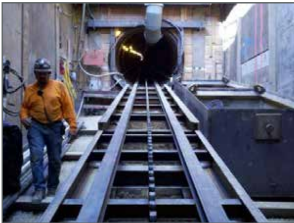
Figure 13. Upper tunnel launch pit just below PVDS/25th Street.
