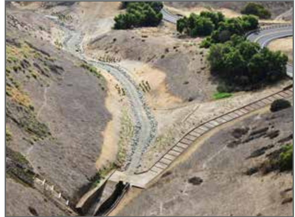
Figure 20. Completed maintenance access to the San Ramon Canyon inlet structure.
