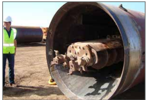
Figure 7. Lower tunnel Rotohead excavator.
