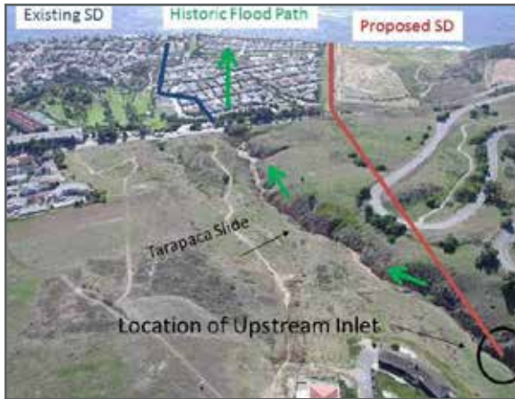
Figure 4. Overview of San Ramon Canyon Storm Drain looking downstream.
