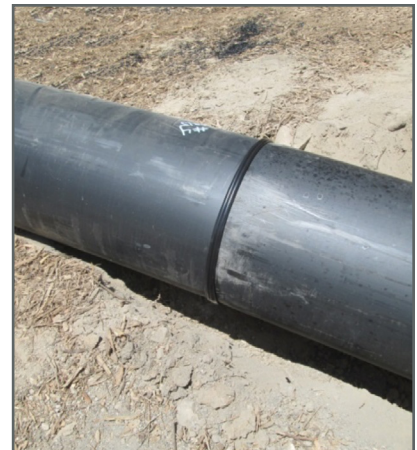
Figure 1: Completed HDPE weld for the Dollar Hill Force Main project.
