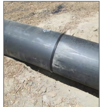
Figure 1: Completed HDPE weld for the Dollar Hill Force Main project.
