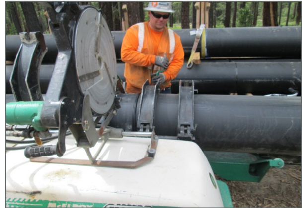
Figure 7: Fusion welding for the NTPUD Dollar Hill Force Main project. This joint is currently in the cooling phase.
