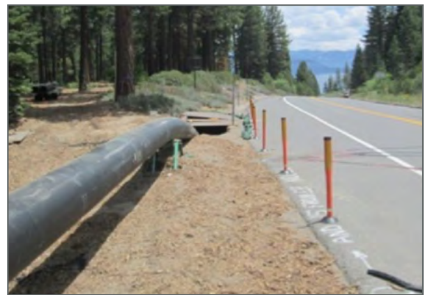
NTPUD Dollar Hill force main project
