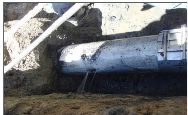
Figure 5: Existing leak in PVC force main
